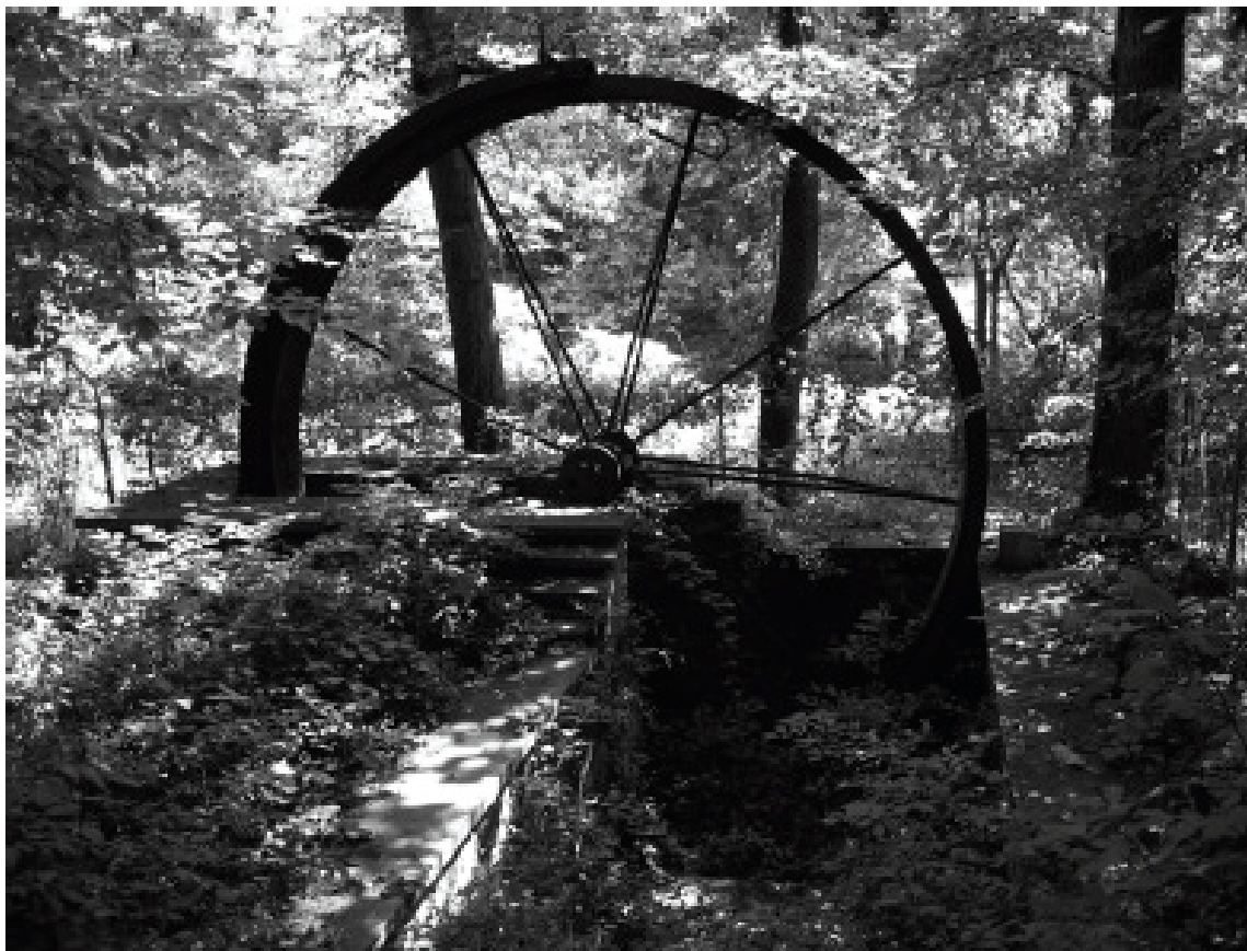
This relic waterwheel is easily accessible the Gwynns Falls Trail. Near the trail is the remnant of a carriage path which provided access to the Orianda Mansion, the ruins of a mock fort (apparently inspired by Winans' years in Russia), and the foundations of old farm structures which were part of the nineteenth-century Crimea estate.
